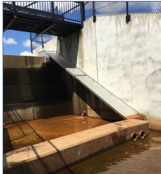
Wyassup Eel Pass. Left: Transverse slope allows the eel pass to operate at varying headpond elevations. This eel pass was incorporated into the design of the dam repair with the entrance of the eel pass secured between the dam's wing-wall and a concrete eel guidance wall. Right: The exit chamber was extended to meet the eel ramp at a lower elevation.
