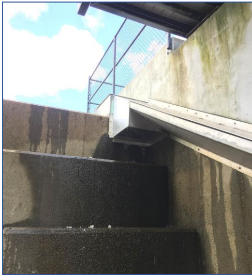
Wyassup Eel Pass. Left: Transverse slope allows the eel pass to operate at varying headpond elevations. This eel pass was incorporated into the design of the dam repair with the entrance of the eel pass secured between the dam's wing-wall and a concrete eel guidance wall. Right: The exit chamber was extended to meet the eel ramp at a lower elevation.
